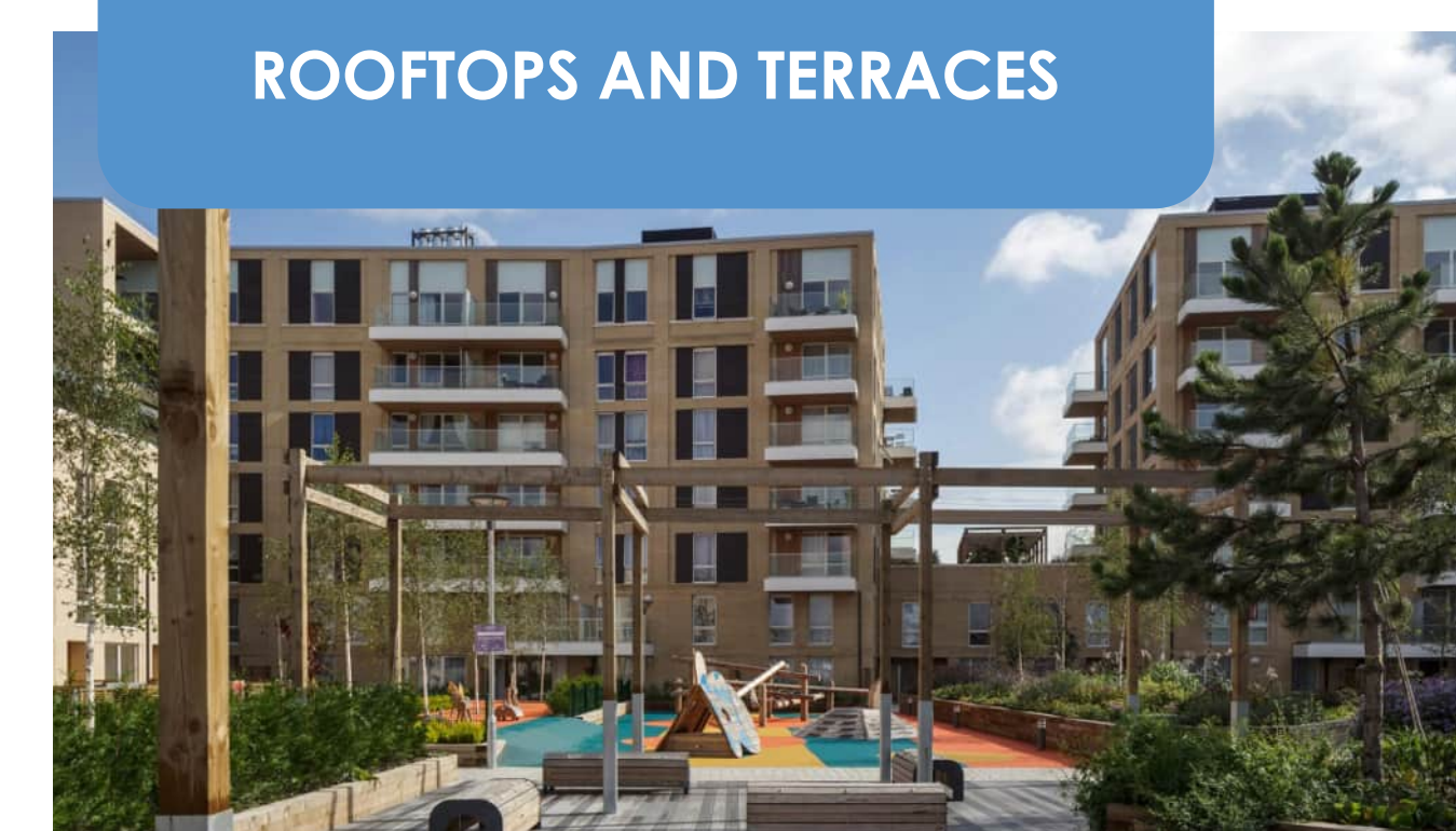
ROOFTOPS AND TERRACES
